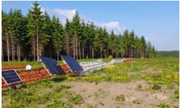
Houdremont wind farm measuring mast vandalized May 2025
