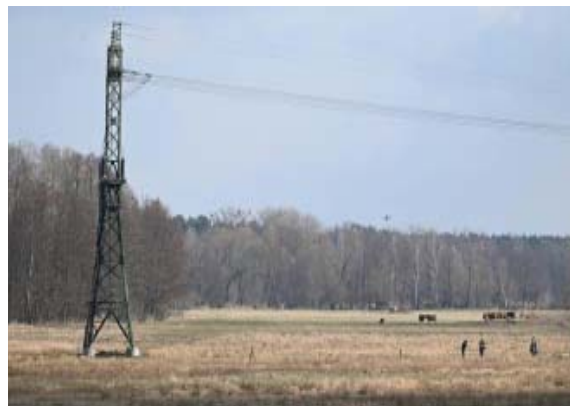
photo:Steinfurt, southeast of Berlin, March 5, 2024. The last pylon of the high-voltage line, burned at the location where the cables run underground to supply the Tesla factory.
